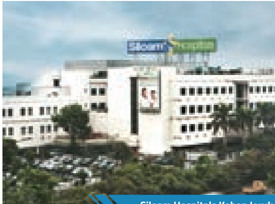
Siloam Hospitals Kebon Jeruk
